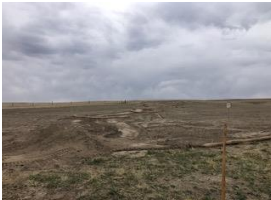
Swale created by skid steer and hand raking the area
