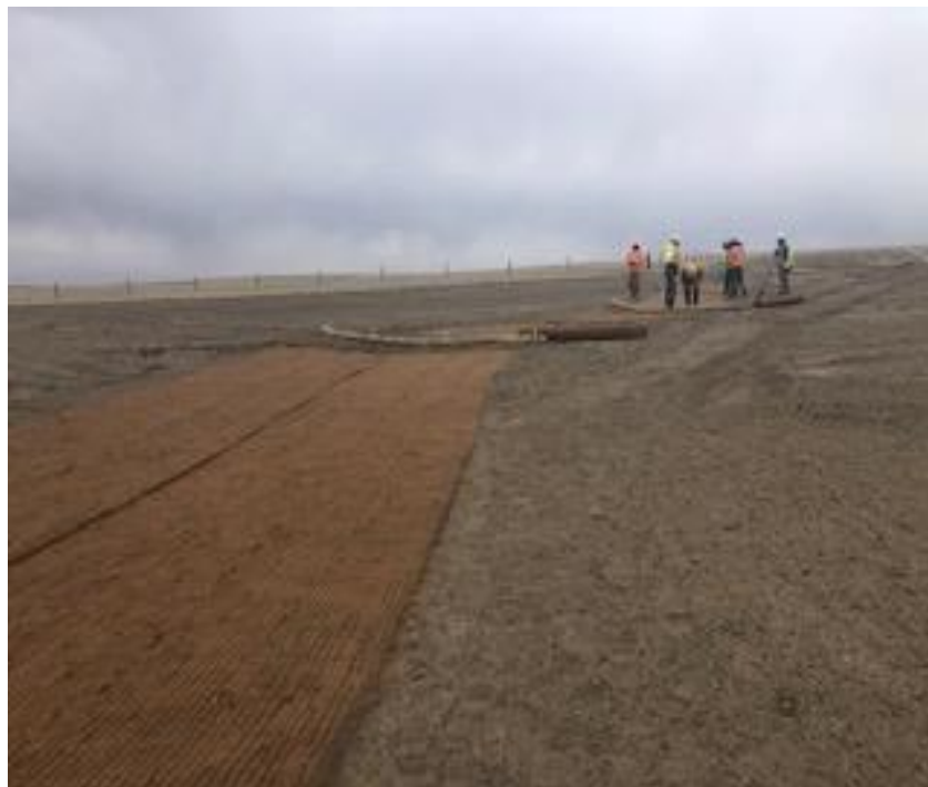
Installing coconut matting over swale area and installing erosion control device
