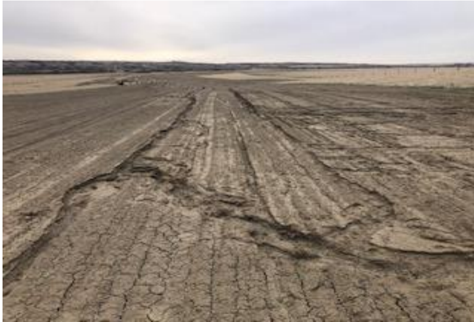
Erosion from run off on right of way
