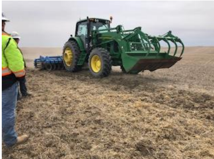
Tractor discing the right of way
